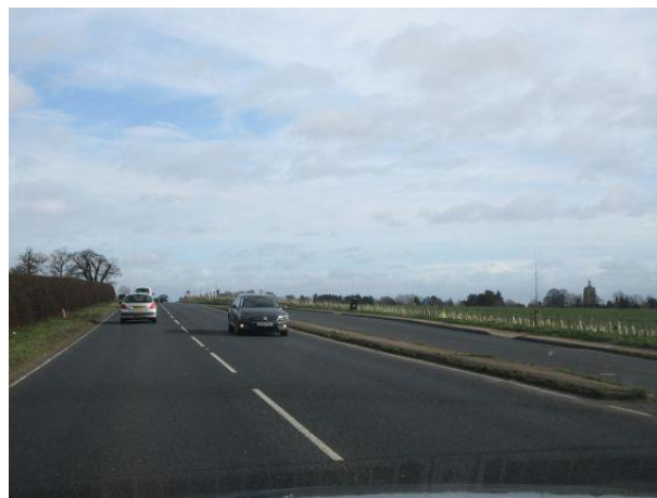
Photograph 22 East on the A47. There are many laybys to use as a potential lay-up area to assist with management of traffic congestion.
