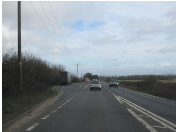
Photograph 21 East on the A47 passing another potential lay up area.
