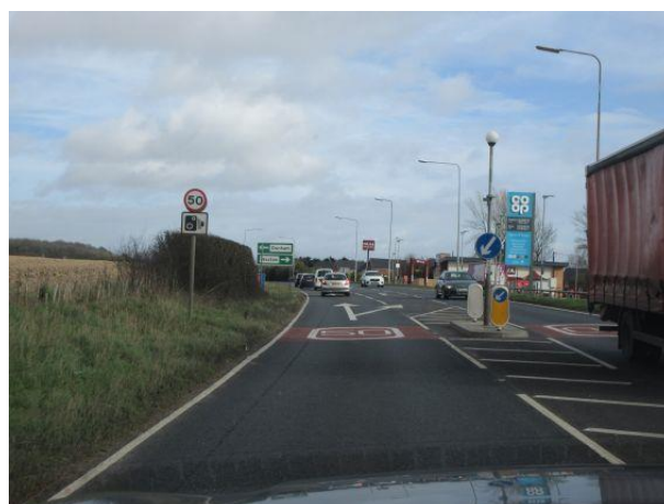
Photograph 23 Traffic calming measures on the A47 at Necton where central island furniture will need to be removed. Vehicle moves away from camera.
