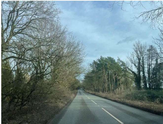
Photograph 38 Dereham Road, vehicle moves away from the camera, negotiable. Tree pruning may be required depending on growth at the time of movement.
